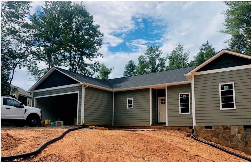
Burke County, NC - new housing construction near Morganton, NC.
