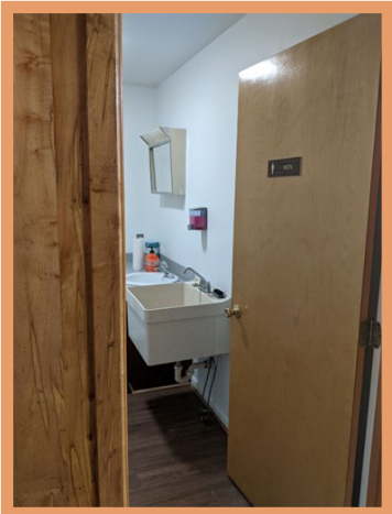
Signage should be in braille and mounted on latch side of door
