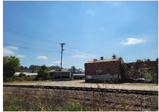
NCDOT Property at Biltmore Village in Asheville, NC
