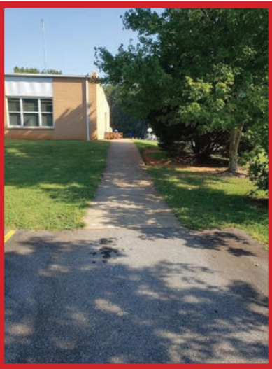
Access routes cannot exceed 2% cross slope.
