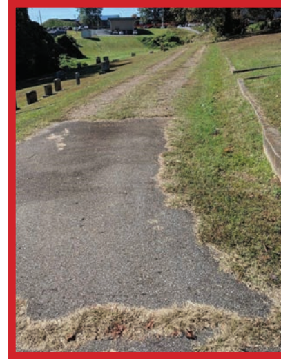
Main roadways should be paved.
