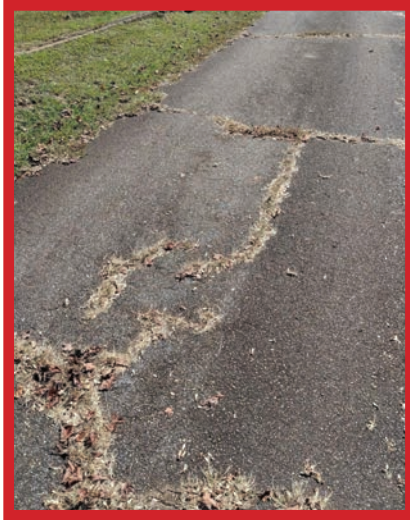
Remove vegetation and reseal pavement.
