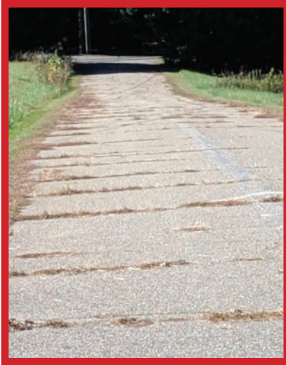
Remove vegetation and reseal pavement.
