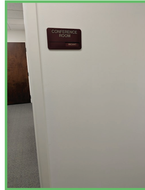
Room signs should be mounted on the wall, on the latch side of the door.
