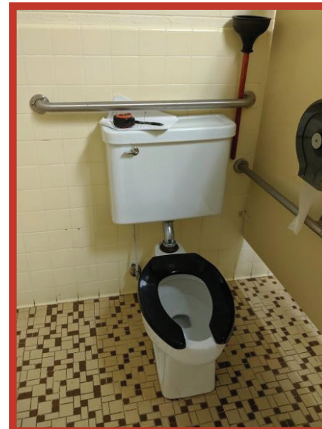
Rear grab bar is too high due to back of toilet.
