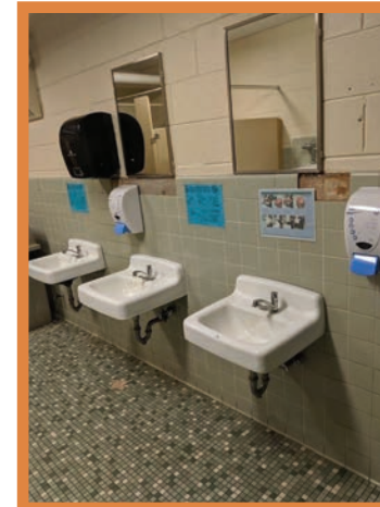
Insulate pipes under sinks and lower mirrors.
