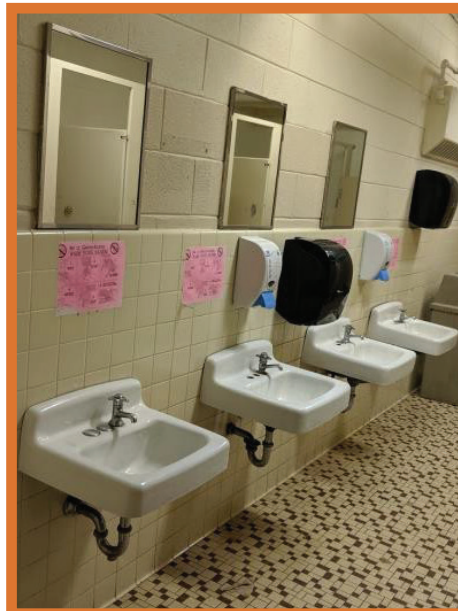
Insulate pipes under sinks and lower mirrors.
