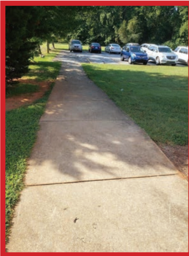
Access routes cannot exceed 2% cross slope.
