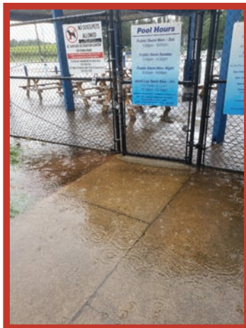
Drainage issues at pool accessible entry.
