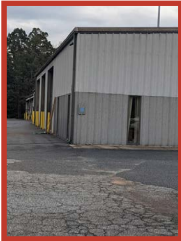
Need designated accessible parking with signage and striped access.
