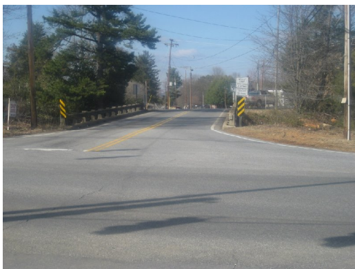
Bridge at Hwy 70 and N. Center Street
