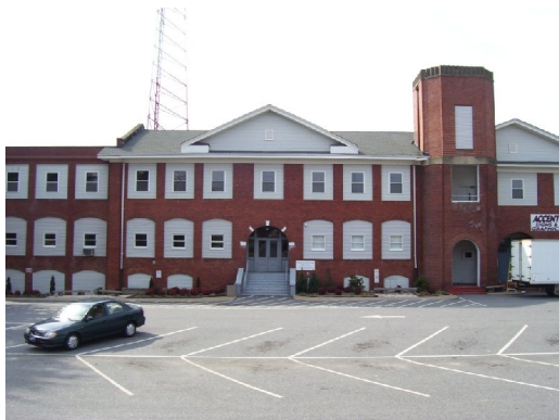
Old school building
