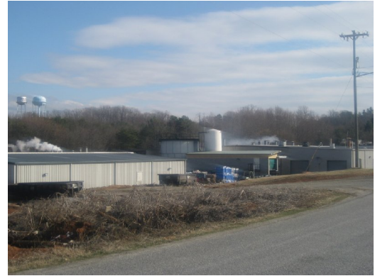
Industrial facility in Cline Industrial Park
